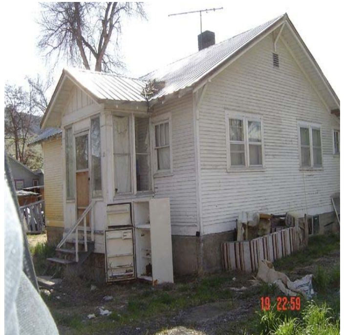
Asbestos house in Dixon, Montana.
