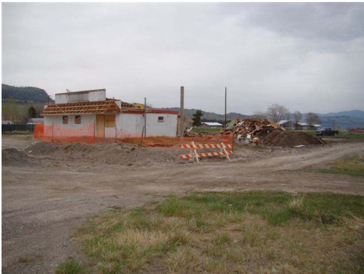
Elmo store before demolition.
